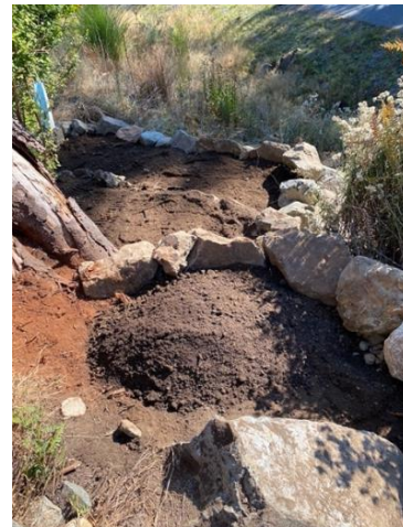
→ Finished terraced beds
