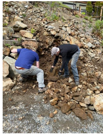
Building the terraces above the road
